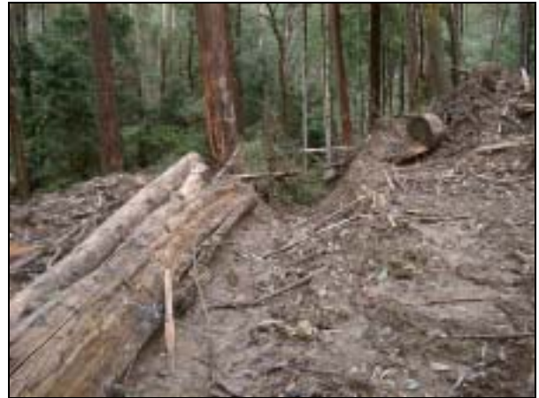
Photo 16. Log removed from temporary culvert on snig track in accordance with Code requirements.
