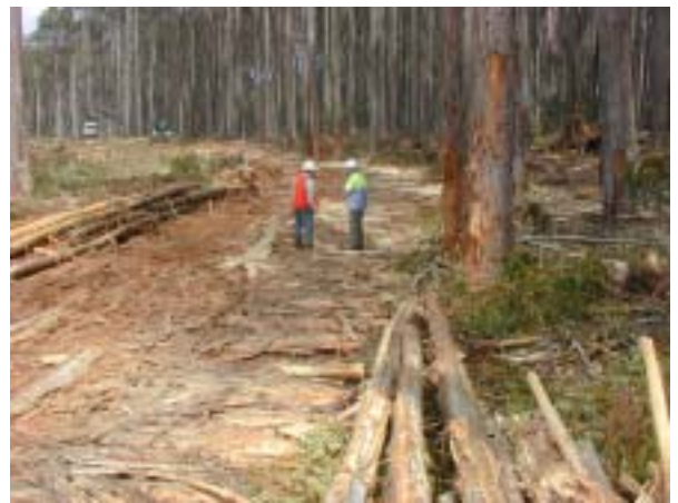
Photo 18. Appearance of a cord and matt snig track during use. There had been no exposure of mineral earth during harvesting within this coupe. (Note: the coupe shown was not part of the audit program.)
