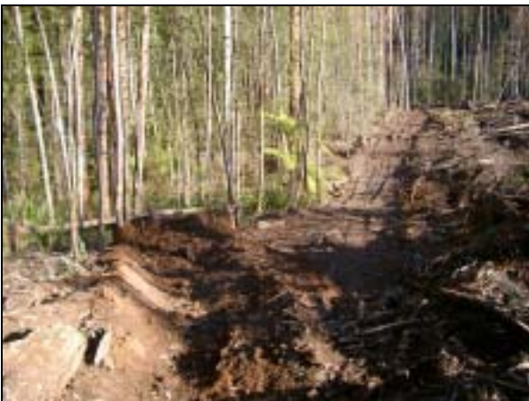
Photo 3. Boundary track with bar and breach pushed beyond coupe boundary.
