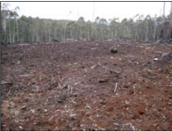
Photo 14. A good example of coupe landing ripping using the beak of an excavator.
