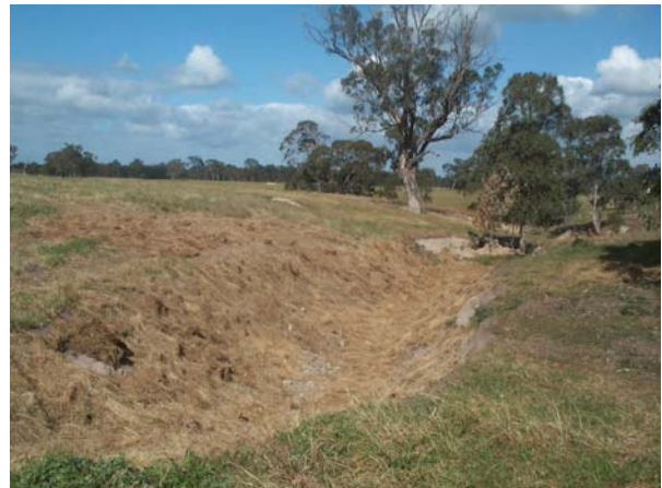
After: Cleared area ready for revegetation.
