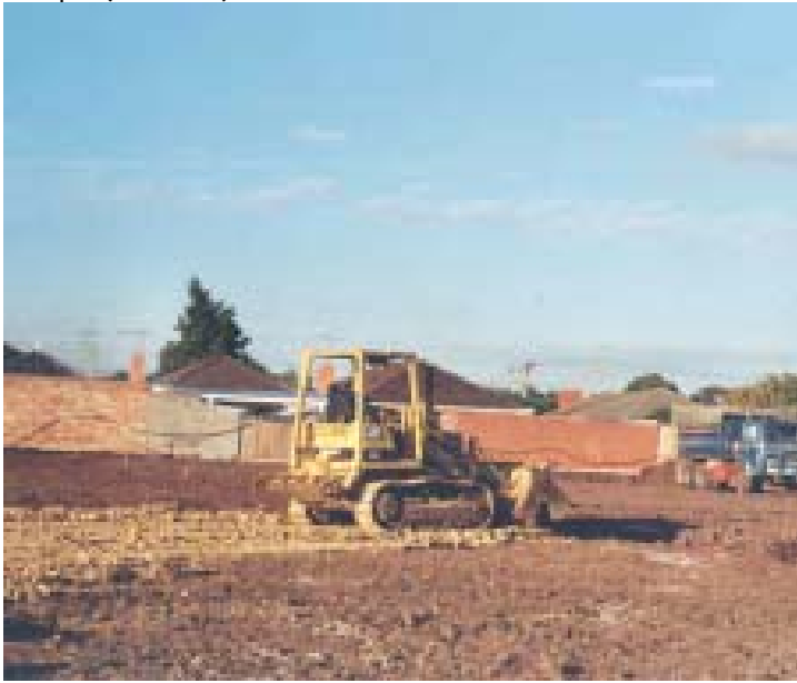
9. Preparing subgrade (forming to starting levels) (6/5/02)
