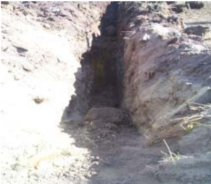
3. Excavation of test pit to identify edge of quarry (10/4/02)
