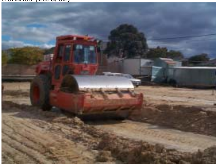
33. Compaction of clay lift using vibrating drum roller (20/8/02)
