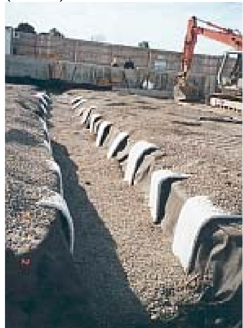
18. Construction of gas ventilation along service trench (31/7/02)
