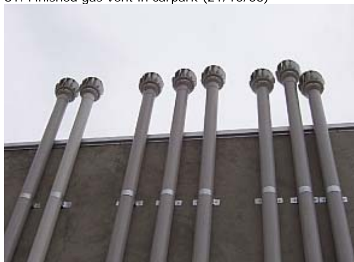
83. Rotary vents connected to gas ventilation layer (21/10/03)
