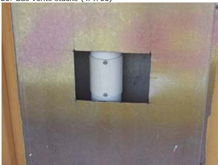
82. Provision for sampling from gas vents from beneath building (21/10/03)
