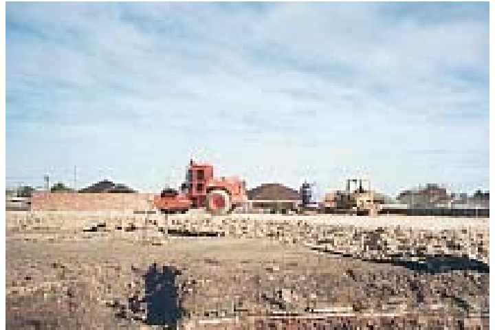
20. Compaction of clay cap (31/7/02)
