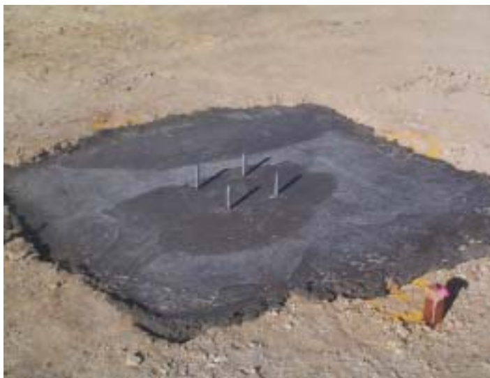
48. Finished pile cap (25/9/02)
