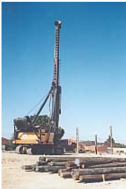
68. Piling rig and timber piles (12/2/03)
