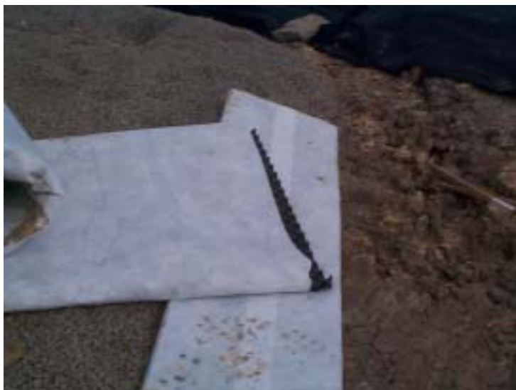
31. Strip drain material used to construct gas vent layer in trenches (20/8/02)
