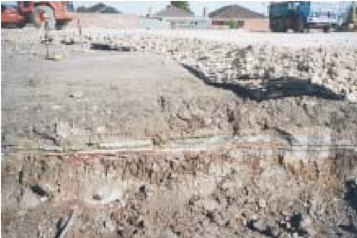
19. Installation of clay cap (including gas vent layer and geosynthetic fabric) (31/7/02)
