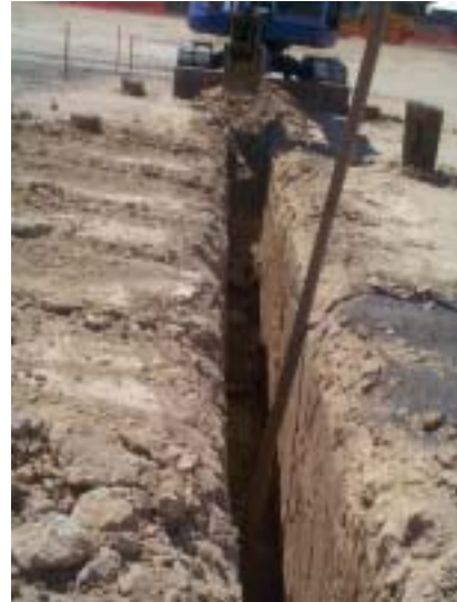
51. Sewer trench being excavated in compacted clay beneath supermarket (14/11/02)
