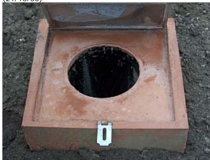
83. Rotary vents connected to gas ventilation layer (21/10/03)
