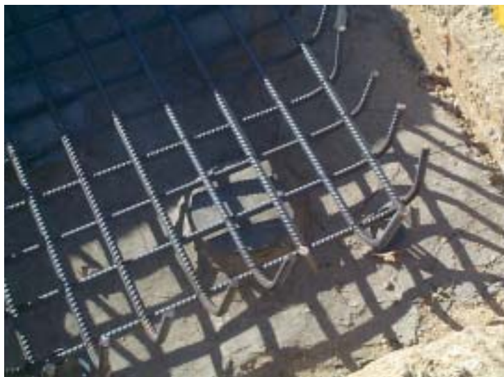
47. Steel reinforcement for pile cap above pile sealed with expanding grout (25/9/02)
