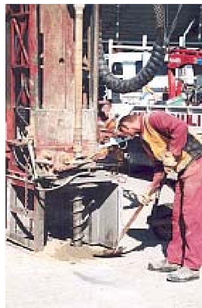
71. Drilling for groundwater monitoring bore within quarry (5/4/03)
