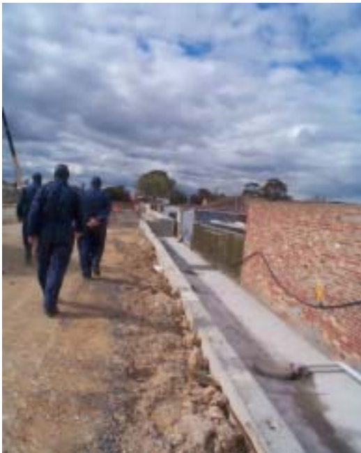
29. Retaining wall, cap and finished surface on southern boundary) (20/8/02)
