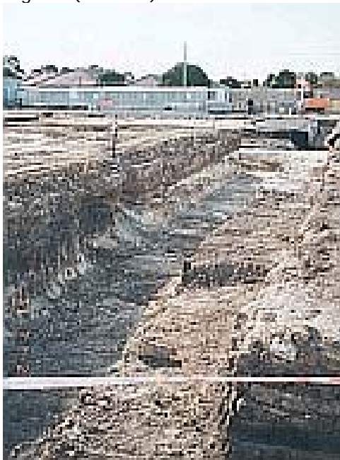
17. Trench excavated to allow clay to be installed around services (31/7/02)
