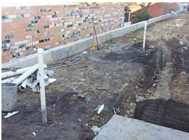
72. Groundwater monitoring bores on southern boundary (11/6/03)
