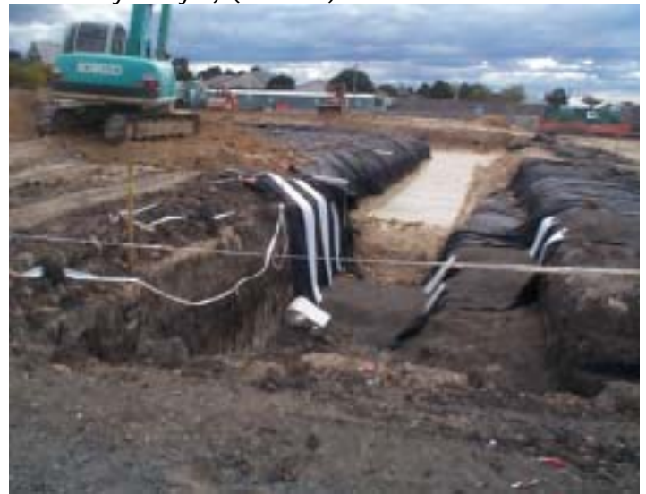
26. Compaction of clay using smooth drum (pad foot roller used to key in layer) (13/8/02)
