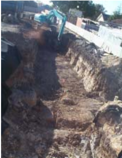
41. Excavation of service trench along southern boundary (25/9/02)
