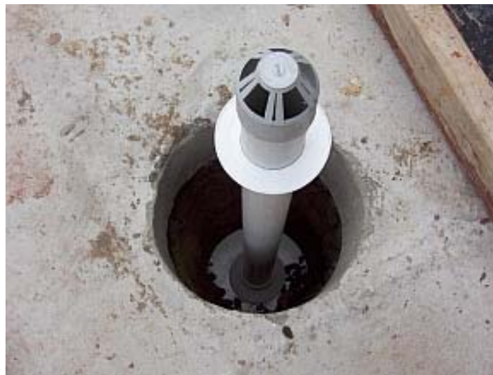
75. Installed gas vent (not sealed) (17/6/03)
