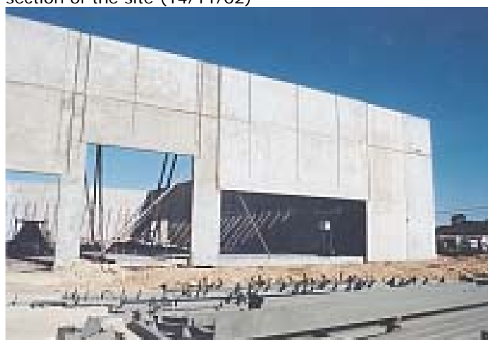
67. Construction of supermarket (12/2/03)
