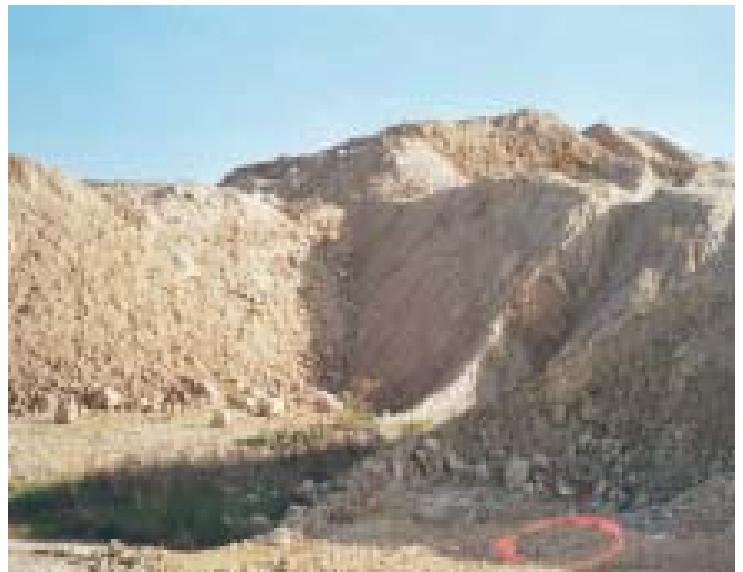
6. Stockpile used for cap construction (6/5/02)
