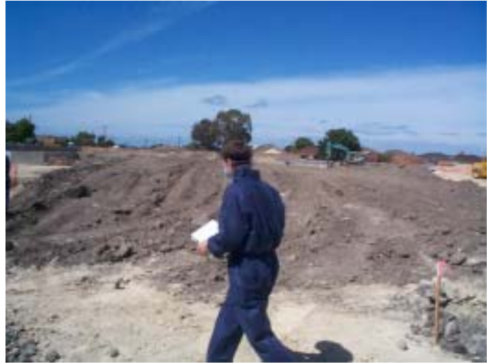
57. Stockpiled contaminated soil from trench excavations (14/11/02)
