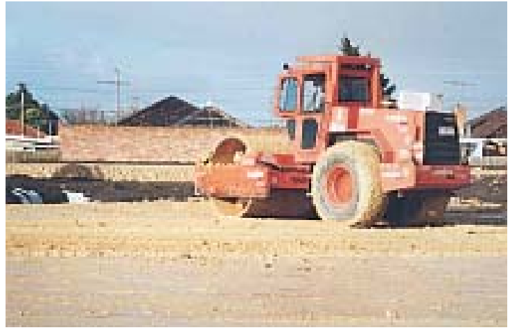
26. Compaction of clay using smooth drum (pad foot roller used to key in layer) (13/8/02)
