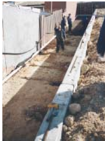
16. Retaining wall and cap construction along southern boundary (31/7/02)
