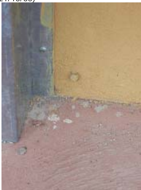
84. Survey point to measure settlement (21/10/03)
