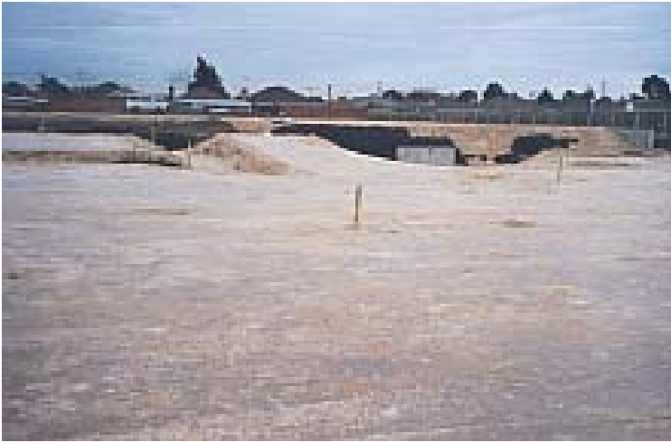
25. Clay capping on western segment of site (9/8/02)
