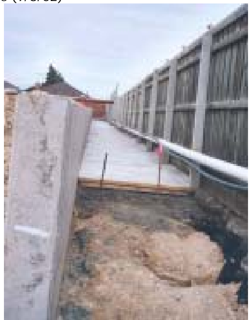
22. Use of strip drain to construct gas vent layer in trenches (9/8/02)
