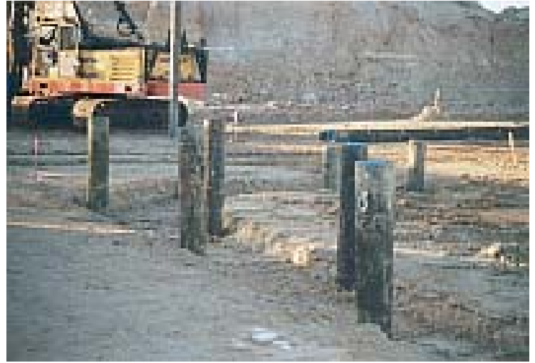
14. Piling for construction of retaining wall along High St (18/6/02)
