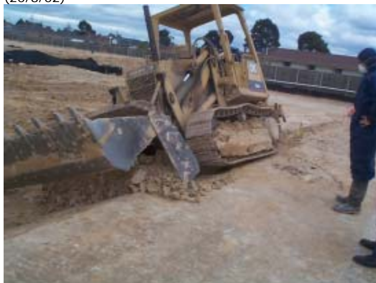
39. Scraping edge of clay layer to check for lamination (20/8/02)
