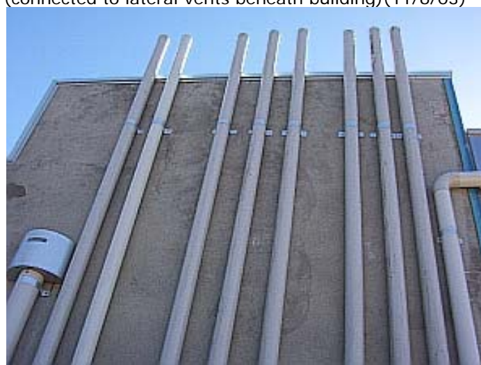
77. Gas vent pipework at rear of specialty shops (connected to lateral vents beneath building) (11/6/03)
