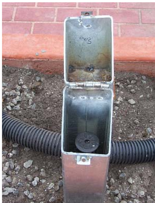
86. Finished groundwater monitoring bore (21/10/03)
