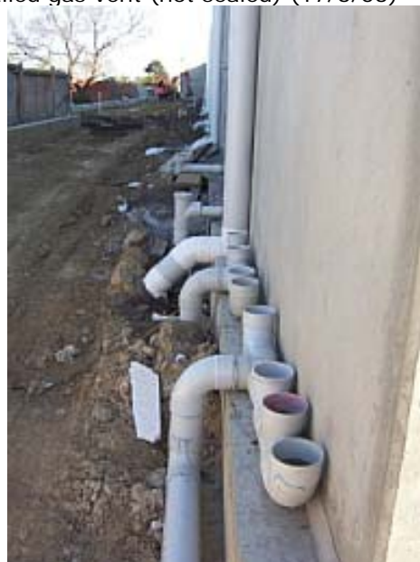
77. Gas vent pipework at rear of specialty shops (connected to lateral vents beneath building) (11/6/03)
