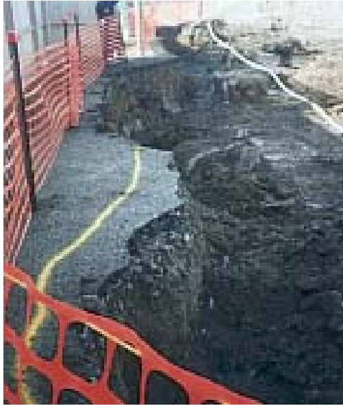
13. Determining quarry edge beneath High St (15/5/02)
