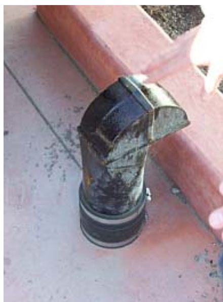
78. Finished gas vent (4/9/03)
