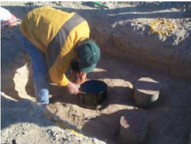
45. Bituminous paint to protect piles (25/9/02)
