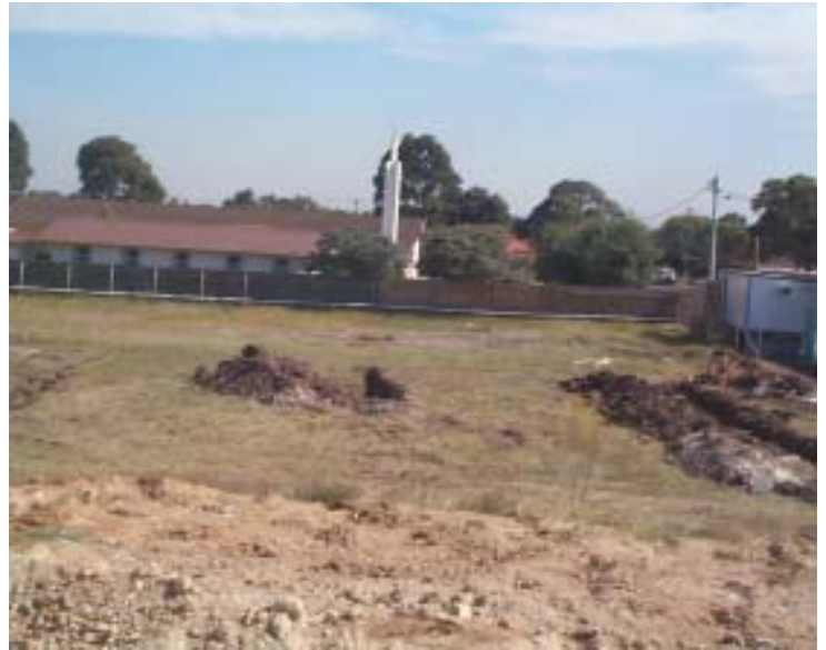
2. Excavation of test pits to identify edge of quarry (10/4/02)
