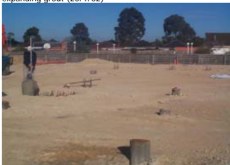
49. Piles beneath supermarket (25/9/02)
