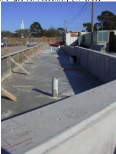
76. Gas vents installed within garden area (4/4/03)
