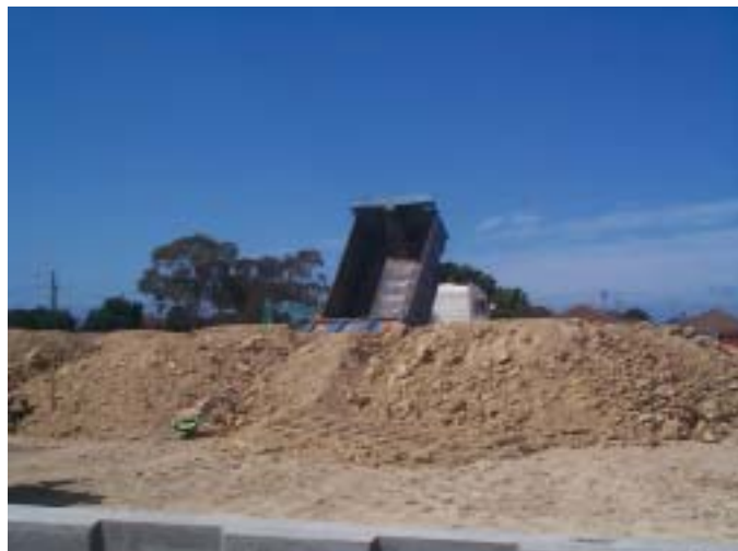
63. Clay from Carlton construction site arriving on-site (14/11/02)
