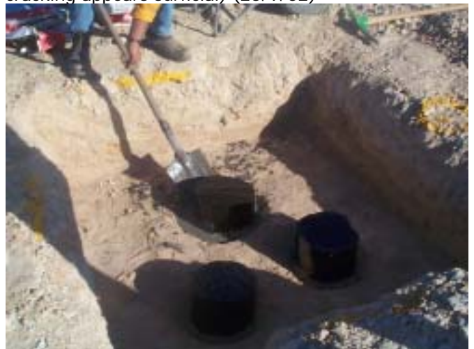
46. Placement of expanding grout around piles to seal gap (25/9/02)
