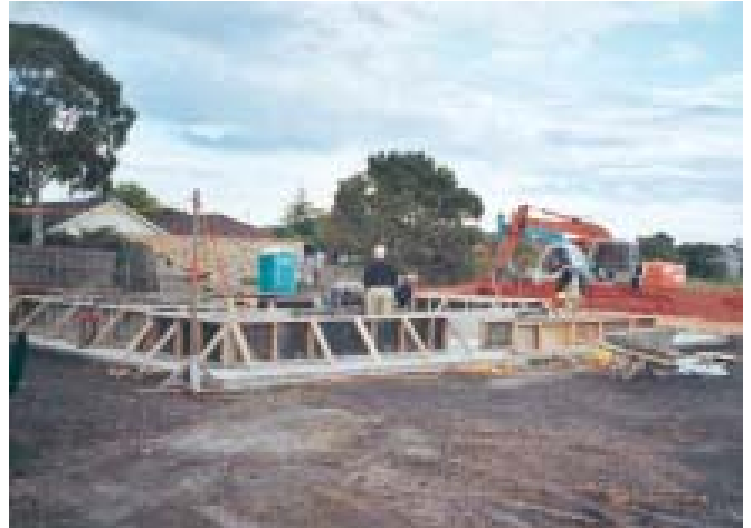
8. Clean area formed for concrete panel fabrication (15/4/02)
