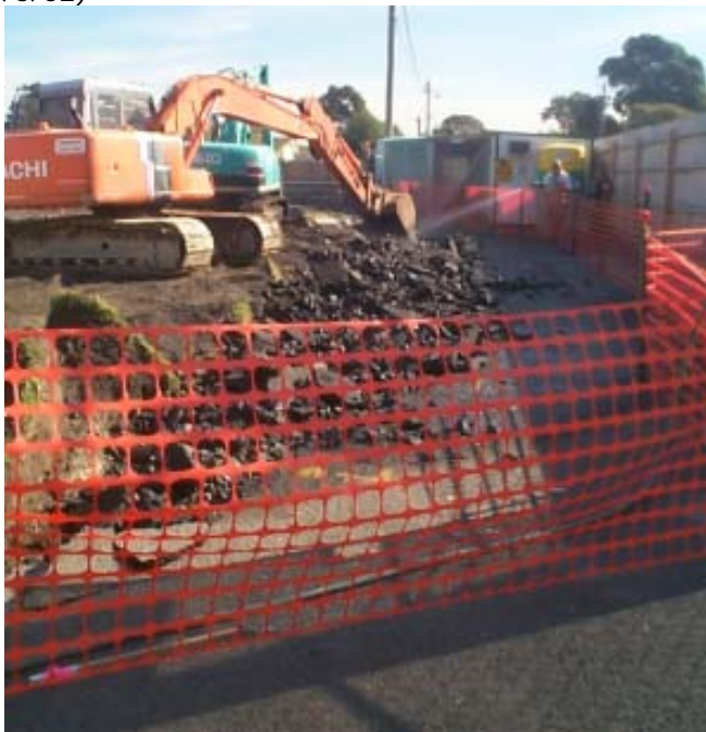
11. Excavation to determine edge of quarry beneath High Street (7 May 2002)
