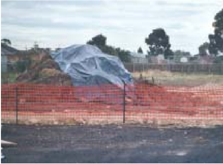
7. Stockpiled vegetation and soil removed during surface scrape (15/4/02)
