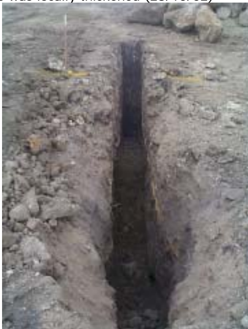
54. Trench to locate quarry edge east of Grid 11 (yellow line marks quarry edge) (28/10/02)
