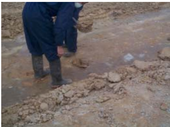
38. Collection of sample of compacted clay for testing (20/8/02)
