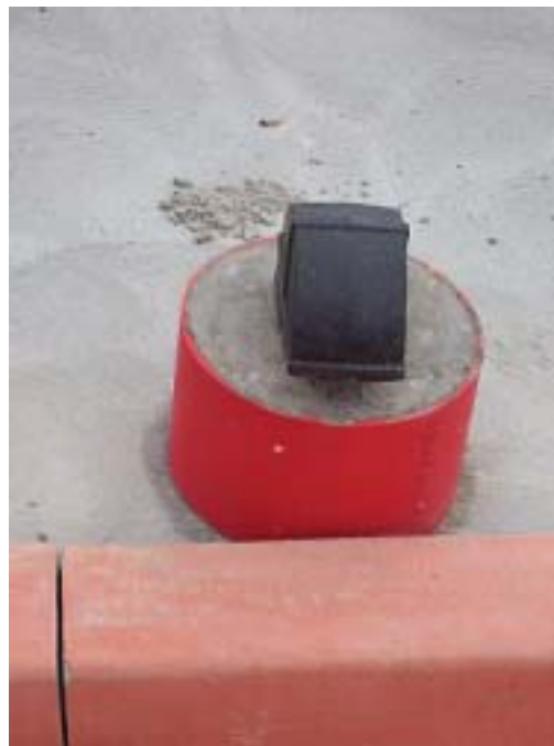
81. Finished gas vent in carpark (21/10/03)
