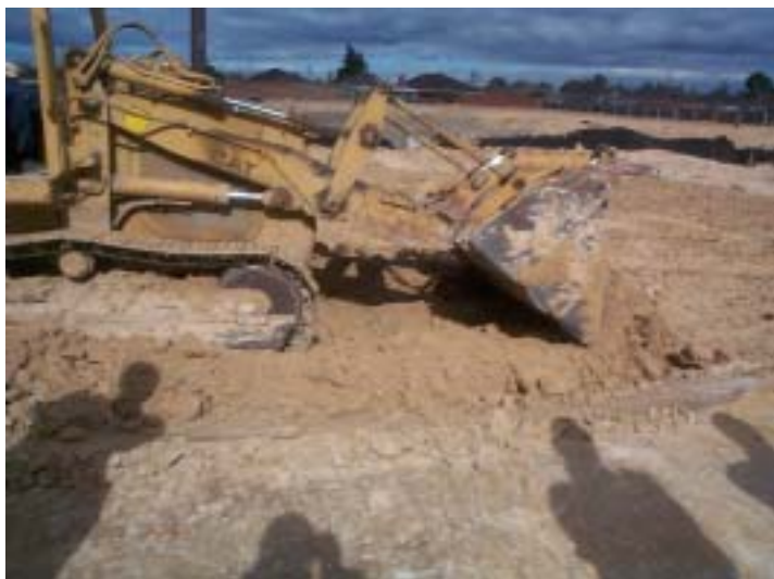
36. Placing next lift of clay for compaction (20/8/02)
