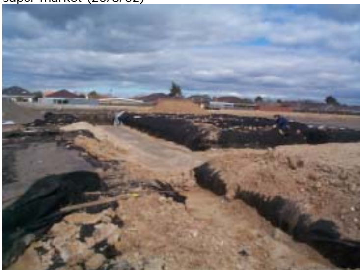
32. Compacted clay within trenches (20/8/02)
