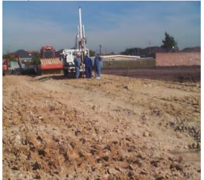
10. Testing of test pad used to confirm performance of clay (7/5/02)
