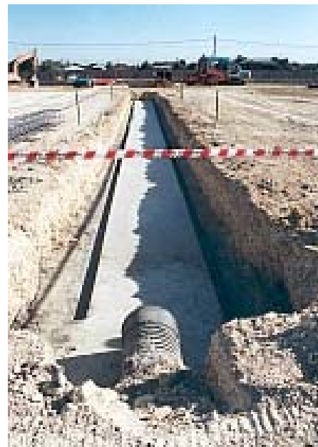
69. Major service trench excavated into thickened clay (12/2/03)
